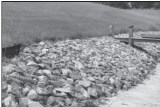
Steep slopes should have woody vegetation replanted.
